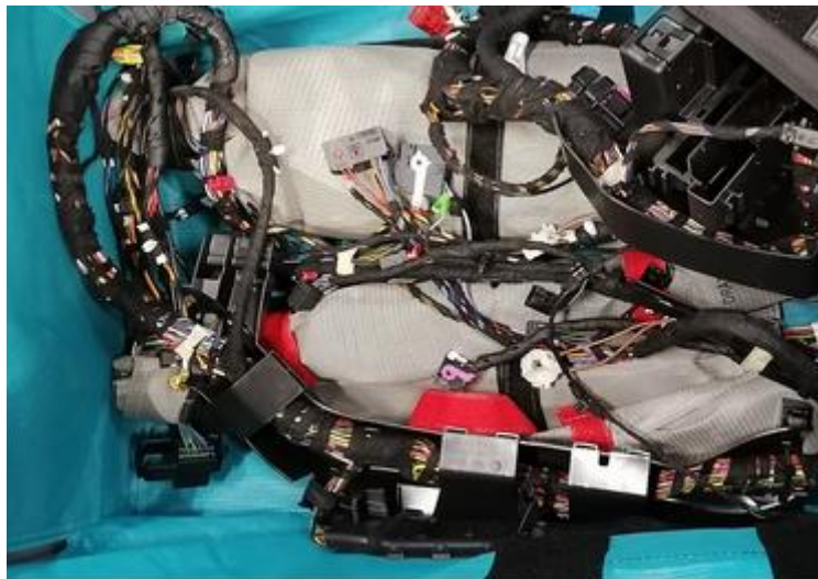
Figure 33. Wiring harness in the transportation box
