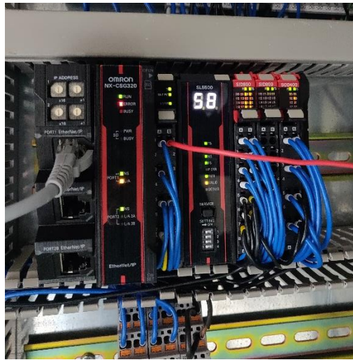
Figure 27. Safety PLC. Its location is shown in Error! Reference source not found.
